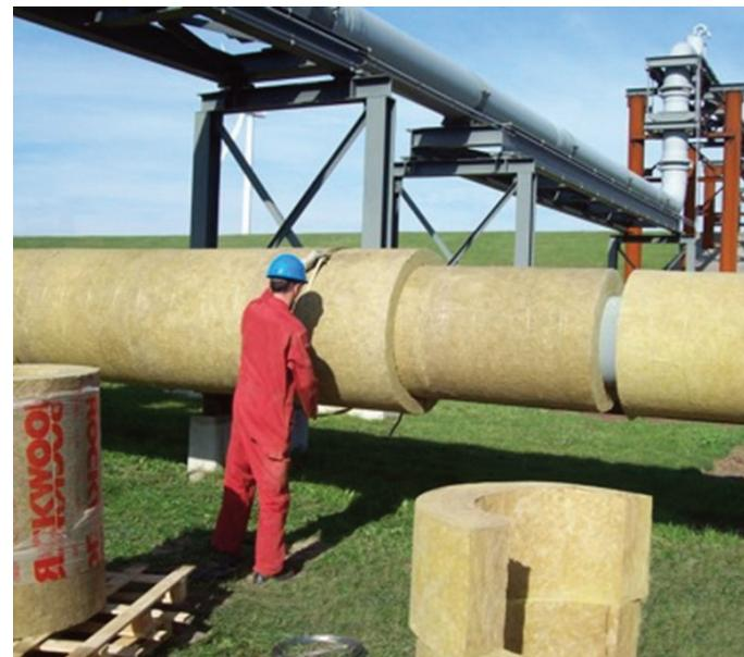
A ROCKWOOL field technician applies ProRox® PS 965 with CR-Tech™ insulation sections in the field. The lightweight, mandrel wound sections apply easily and efficiently, with minimal downtime and safety risks.
