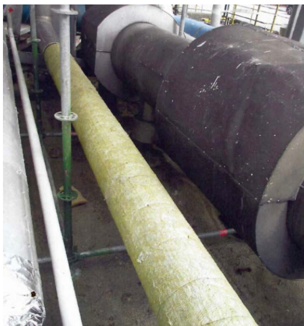
Figure 2. ProRox PS 960 with WR-Tech installed easily and quickly, even on tight clearance areas of the test pipe.
