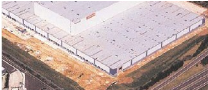
IKEA Distribution centre, Doncaster. DuoRock (plain) roofing board. 80,000m 2
