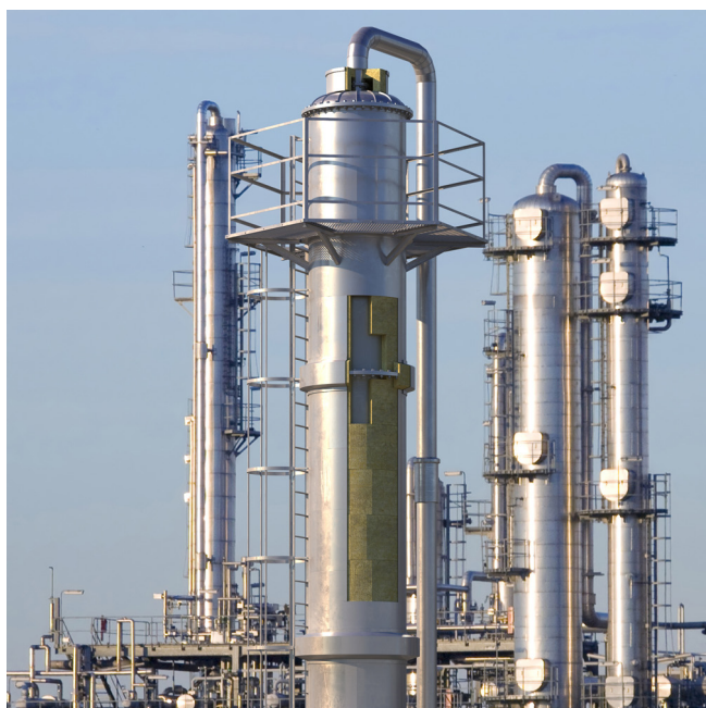
Figure 1. ProRox™ MA 960 with WR-Tech™ can be installed around large columns, tanks, and other equipment to minimise corrosion risks for high temperature applications.
